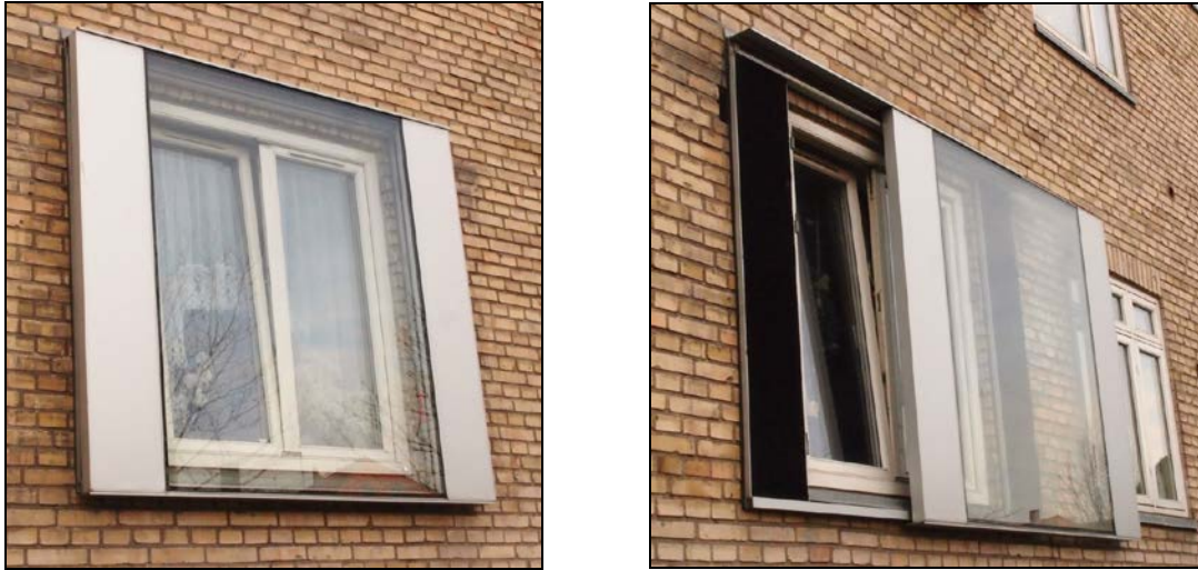
Fig. 3 – Housing in Folehaven. Left photo shows the sound shutter closed, and the photo to the right the open sound shutter. At both photos, the window is open (tilted inwards). An air photo is seen here (press top arrow to see the facade with the sound shutters).
