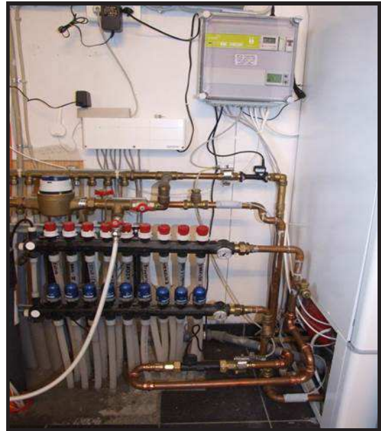
Fig. 2. One of the 54 domestic heat pumps subsequently installed with sensors and actuator that can be accessed over an Internet connection.
