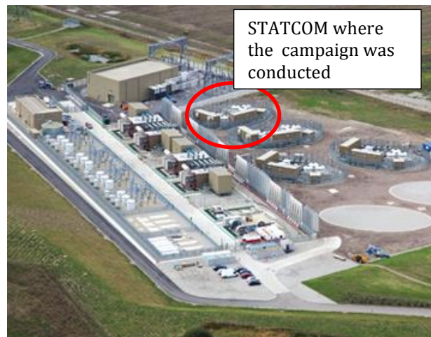
b) Photo of Clevehill substation, where the voltage on the four circuits of LAOWPP01 is being transformed from 150 to 400 kV. Photo is adapted and modified from [116].
