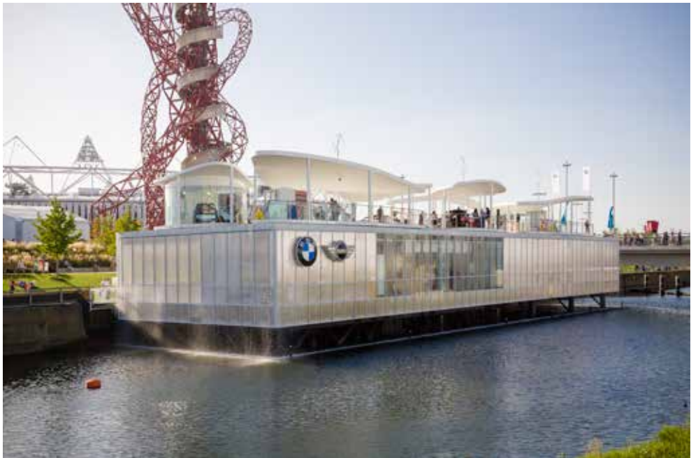
Figure 7-8: 7) BMW Pavilion, London 2012 Olympic Park – Digital fabrication drawings 8) Finished Pavillon.
