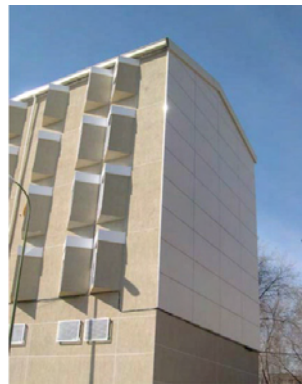
Figure 14 – Rehabilitated building – North and East façades
