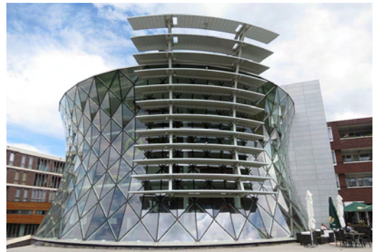
Figure 8 – The energy station is situated in the basement of the the Gen Coel building, Heerlerheide Centrum (HHC)
