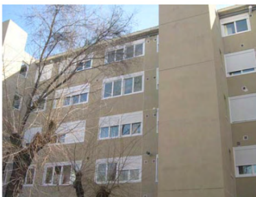
Figure 15 – Rehabilitated building – West façades
