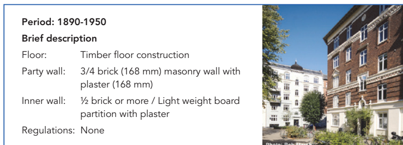
Figure 5.16. Brief description of building type commonly used up to 1950. The photo shows a typical type of building from this period.
