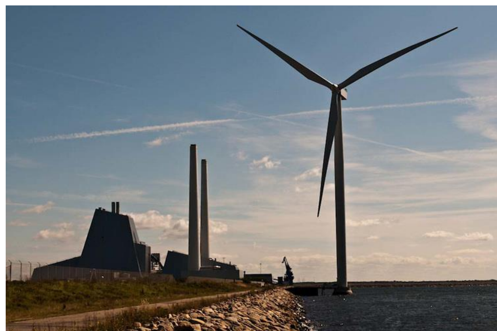
Fig 1. Photo of the Avedøre (Biomass and coal) CHP plant and wind turbine near Copenhagen [1]
