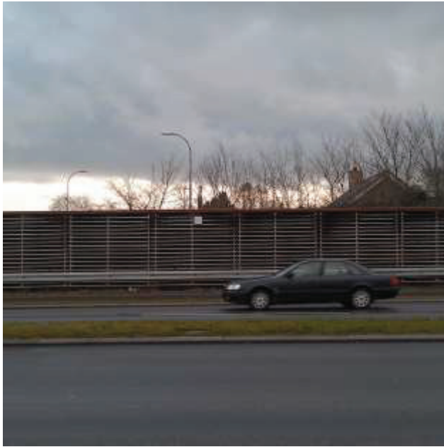
Figure 2-1. The Bluetooth sensor installed on the noise barrier at Grenåvej-Ellebjergvej
