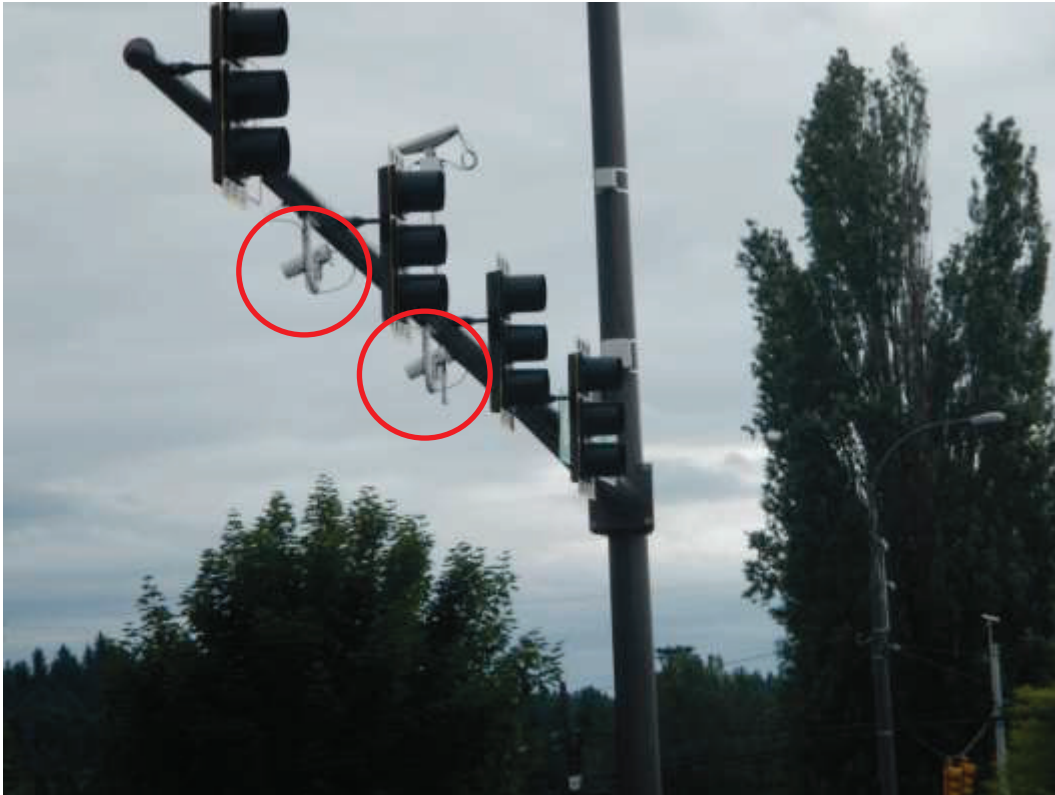
Figure III-6. Pips P327 Spike ANPR sensor
