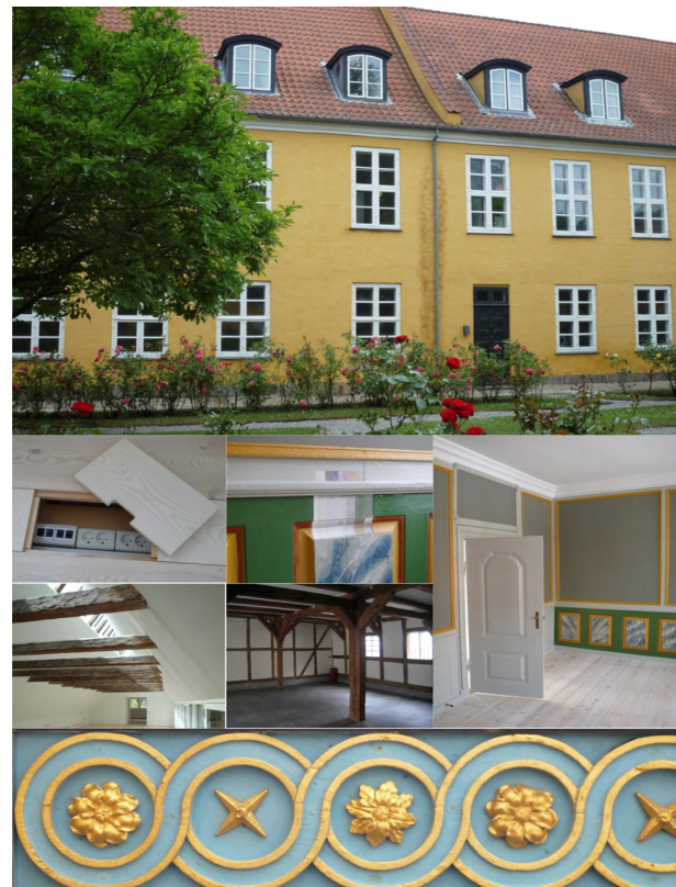
Fig. 8 Photos of the refurbished listed complex, Fæstningens Materialgård.
