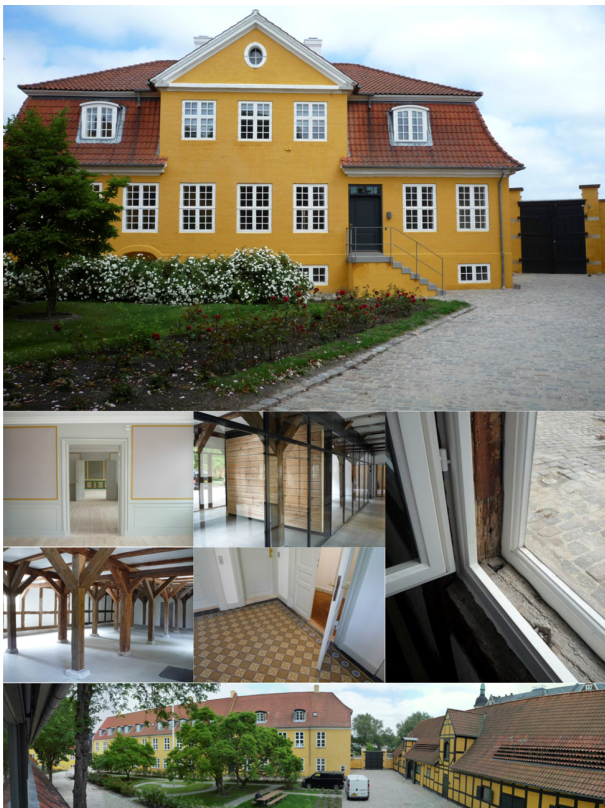
Fig. 7 Photos of the refurbished listed complex, Fæstningens Materialgård.
