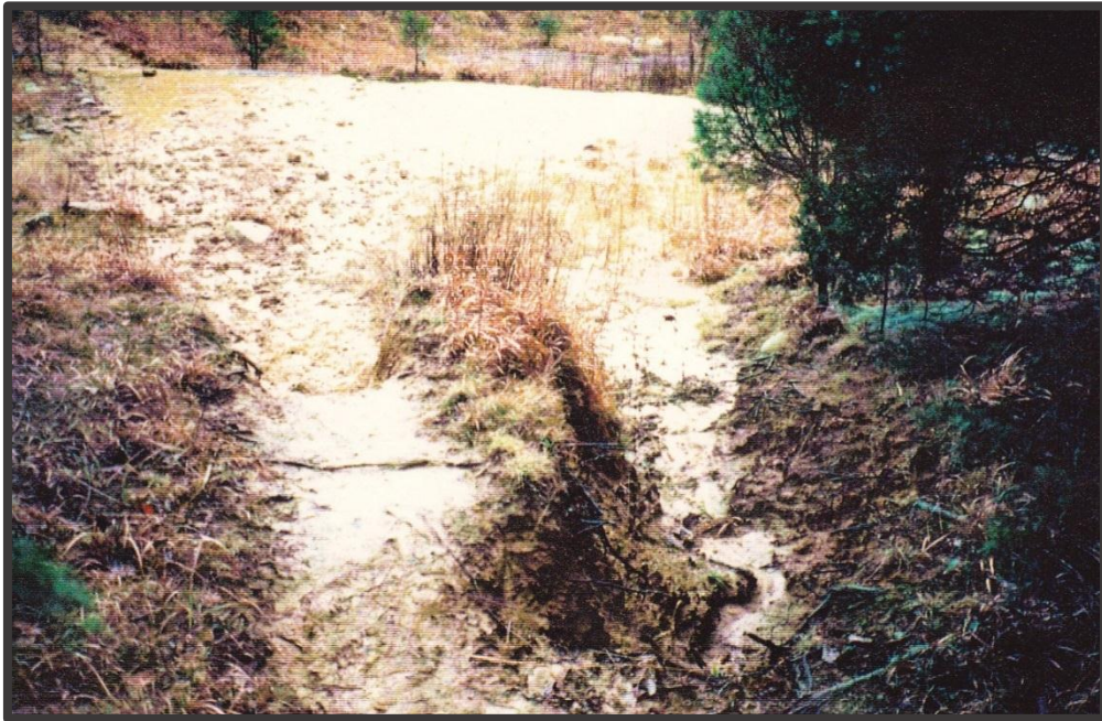
Figure 19: a section of trail during the winter (the wet season). All of the tan color from the left to the right of the photo is liquid mud.
