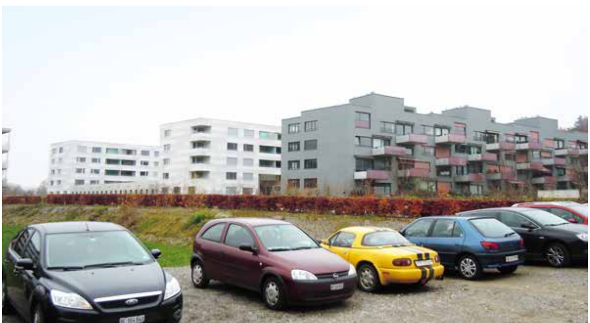
FIGURE 23+24: Above: The light rail is integrated at the new Shopping Centre Westside at the new square Gilberte-de-Courgenay-Platz where there is also a regional train stop -This is the new transit station, leisure and meeting place in Bern West. (Source News.ch 11/12 -2010 Photo: Sam Bosshard) Below: Views to the new quarter Brünnen (Photo by author).
