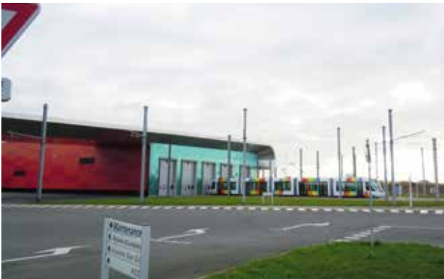
FIGURE 17: As every other element in the Angers light rail project the depot is also thoroughly designed. The building is designed as the wing of an aeroplane, because of the history of the area, which used to be an old airport, the price was 22 mio. euro. (Photo by author).
