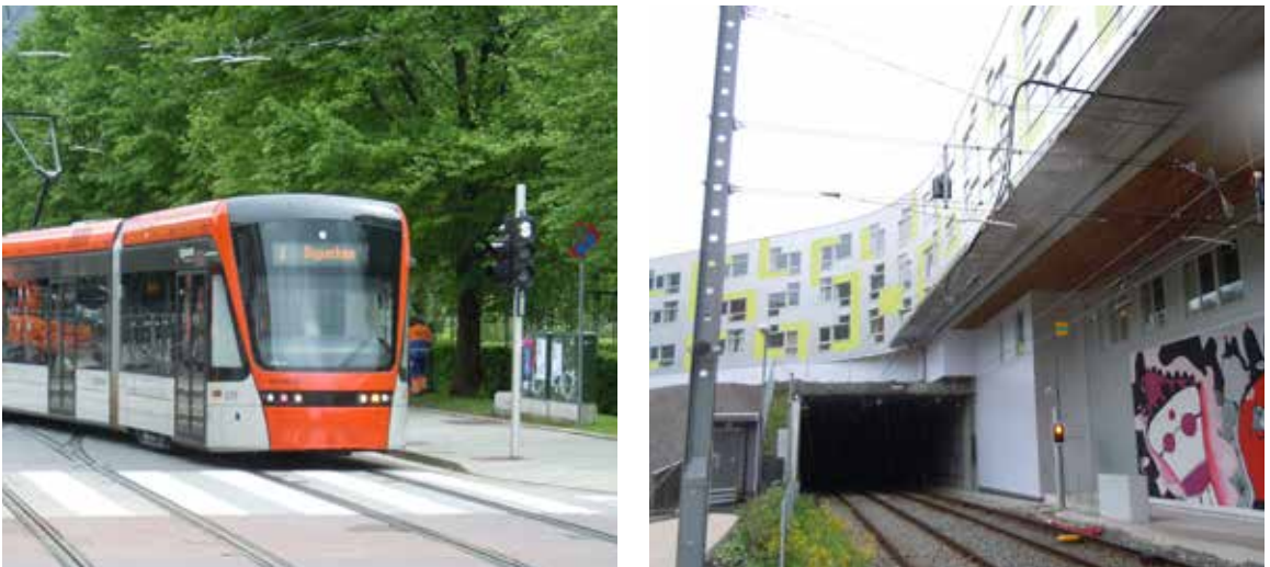
Figure 4: The light rail in Bergen operates in-between the old tramway on the main street in the urban part of the city (left), and as a suburban train shifting to traditional heavy railway tracks in the suburban part of the city, where it is segregated from the urban environment (right). The picture to the left shows the new student housing district Fantoft; the light railscape has been an active part in (re)defining and giving this area a “young identity” with modern art at the light rail node. (Photo by author).
