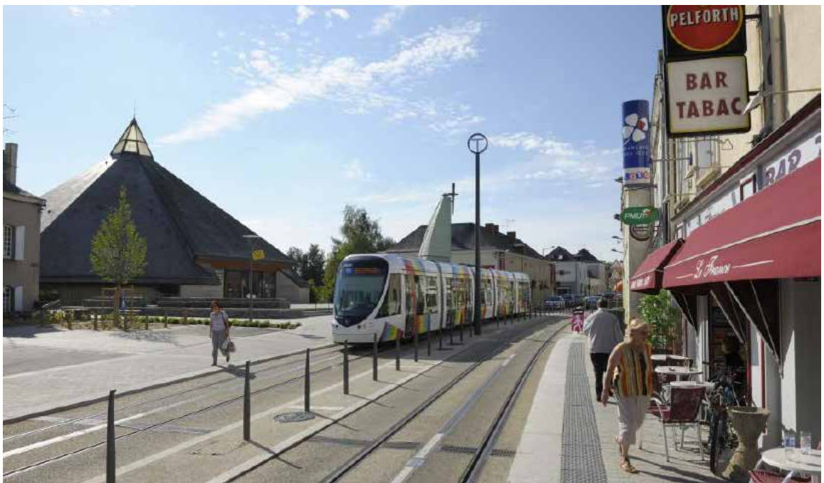
FIGURE 20+21: Avrillé centre before and after the implementation of the Light Rail. Picture from St. Gilles station (Angers Loire Metropole (2012))
