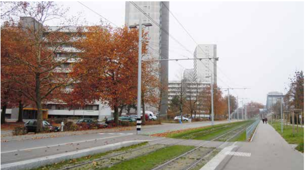
FIGURE 1+2: First impressions of Bern light rail. Above: the central node at the rail way station where the light rail network integrates with the regional network. The roof is shapes like a wave connecting the nodes. Below: The new light rail corridor in the midernistic housing area in Bern West (Photos by author).
