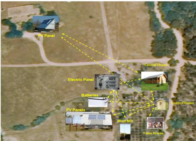
Fig. 11. Wide area view of the Mas Roig Microgrid, Girona, Catalonia,
