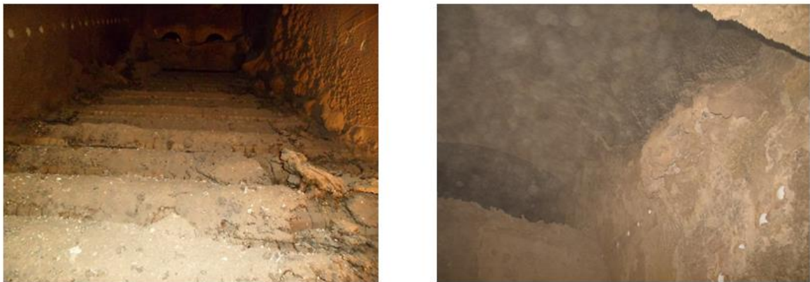
Figure 11: Melted slag on refractory walls.
