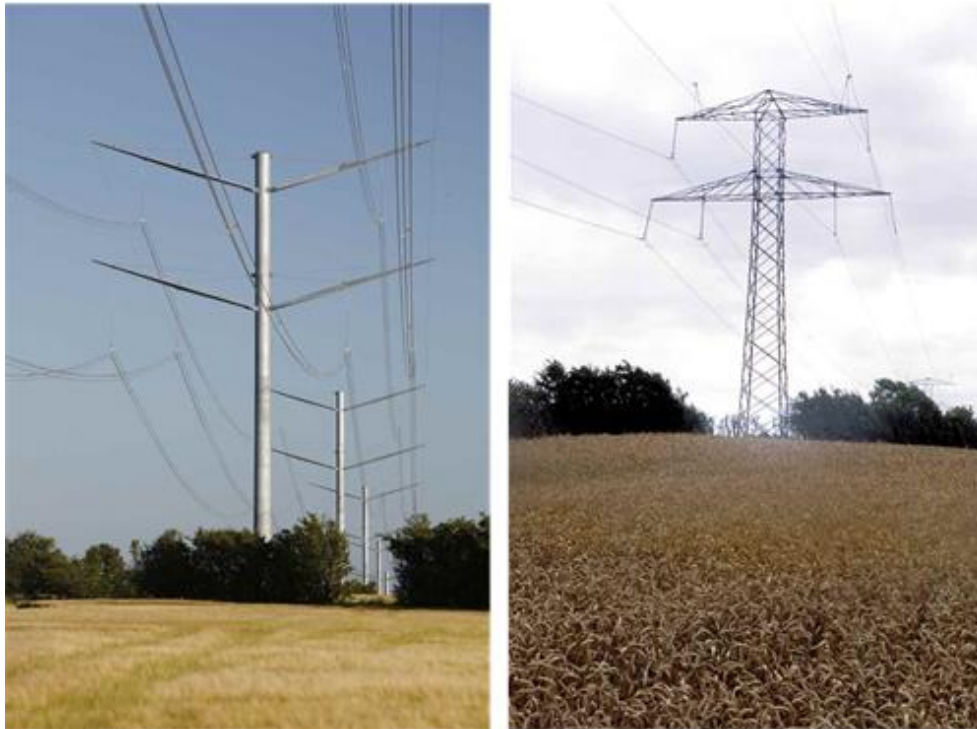
Figure 8 : A picture of the Eagle and the Donau pylons.
