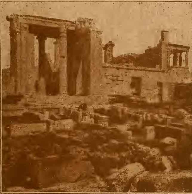
THE ERECHTHEUM FROM THE WEST.
