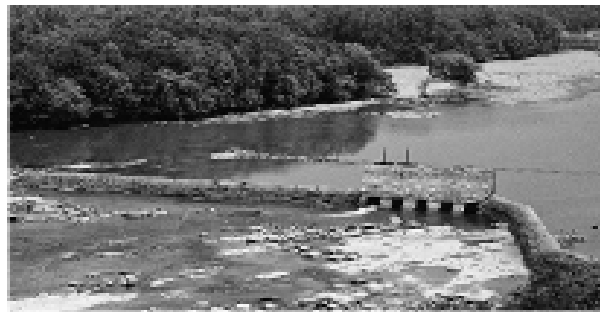
Figure 4. Low-head run-of-river dam on the Savannah River near Augusta, Georgia, a significant blockage for fish passage. Source: U.S. Library of Congress, Historic American Buildings Survey, Historic American Engineering Record.
