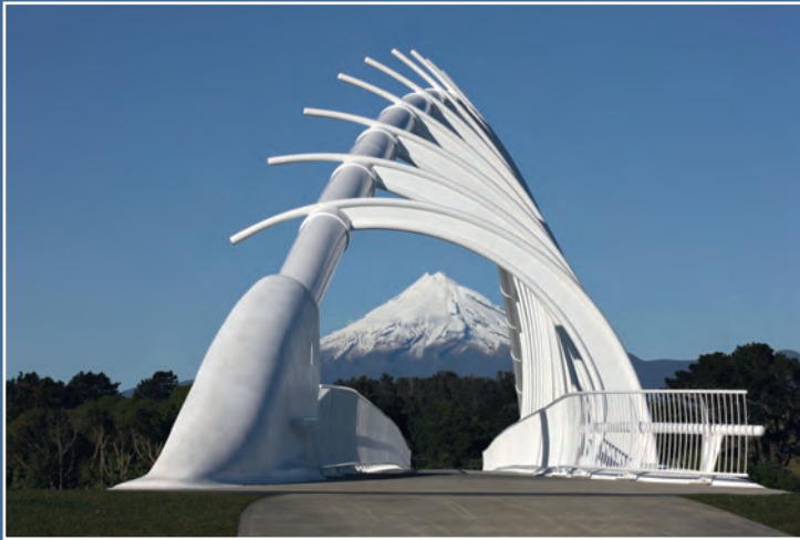
Cover photo: Te Rewa Rewa Bridge, New Plymouth, New Zealand. Courtesy Rob Tucker.
