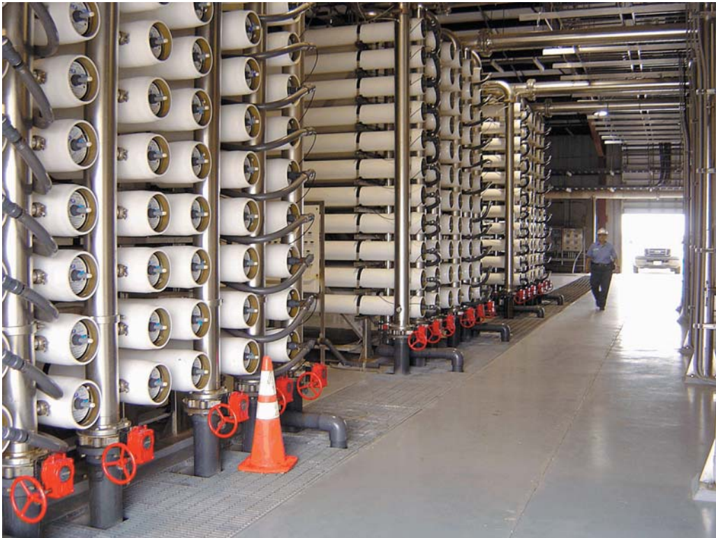
Figure 2. Three banks of pressure vessels (6:11 array each) at the Southmost facility, 2007 (Sturdivant 2007).
