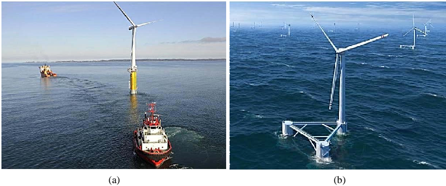
Figure 1.2: Examples of floating wind turbines. The Hywind Demo (a) is a 2.3 MW Siemens wind turbine mounted on a spar buoy foundation. The Windfloat (b) is a 2 MW Vestas wind turbine mounted on a semi-submersible foundation.
