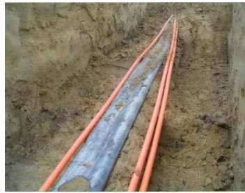
Figure 2. Collapse because of low internal pressure and soil pres.
