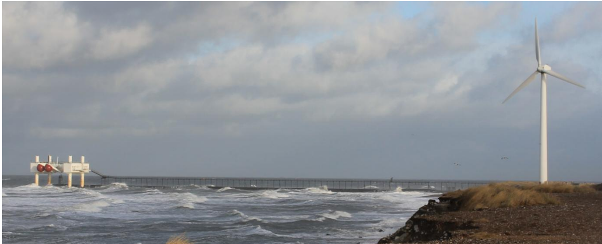
Figure 100. Wavestar (on storm protection mode) and Folkecenter wind turbine at Hanstholm, Denmark.
