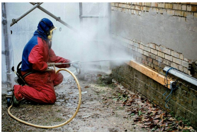
Fig. 7. Water-jet for cutting joints in walls. Cutting is possible especially in interior walls of moderate thickness. However, it is difficult/not possible to make a linear cut.
