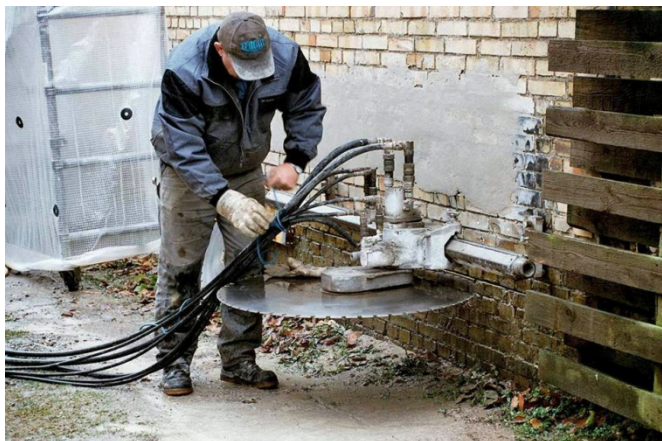
Fig. 5. Circular saw with 1.2 m diameter and diamond tipped teeth. Large excavations around the basement are needed and this together with safety precautions makes the method less desirable.
