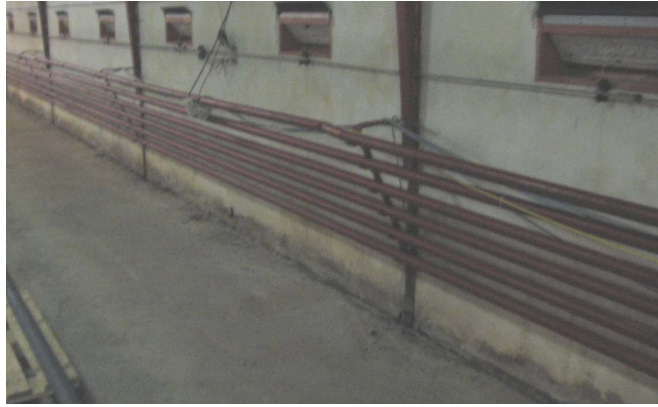
Figure 2.3: The heating system for the stable which is installed on the west and east indoor space of the stable.
