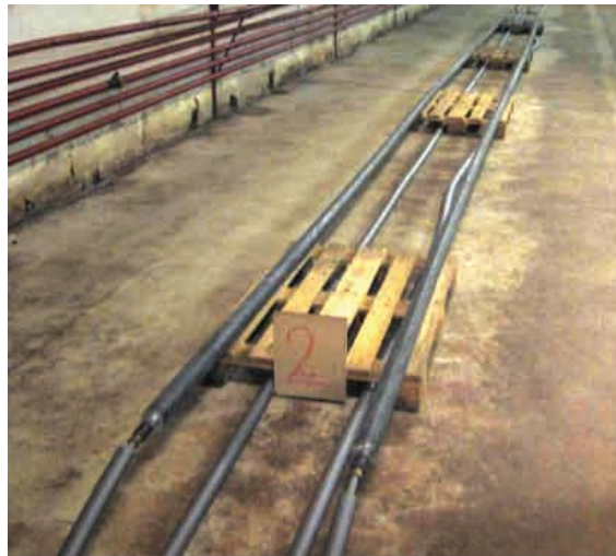
Figure 2.5: The heating system for the animal which is installed 10 cm top of the floor for each zone of the stable.
