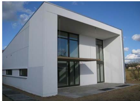
Figure 3.15: Solar shading in house 45.
