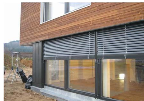
Figure 3.13: Solar shading in house 43.
