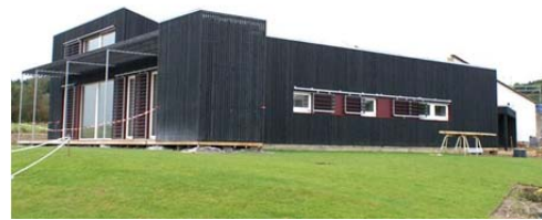
Figure 5.14: Windows in east facade, house 39. Measurements made in room behind the window in the middle in the east facade.
