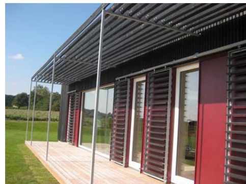
Figure 3.11: Solar shading in house 39.
