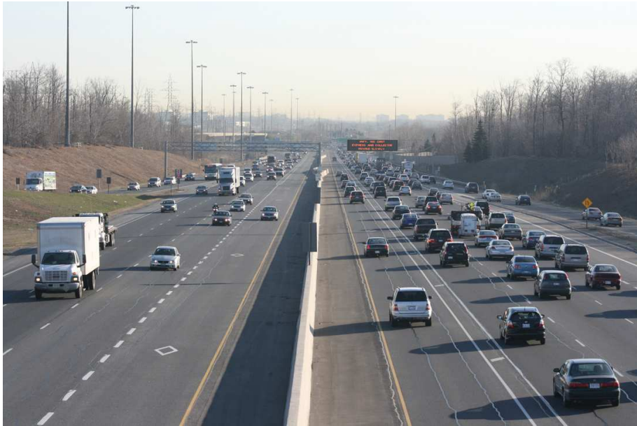
Highway 403 traverses the middle and western edge of Mississauga. Notice the 'diamond' inner lanes, which are high occupancy vehicle (HOV) lanes where cars must have at least a driver and passenger. Photo: Christian Fisker
