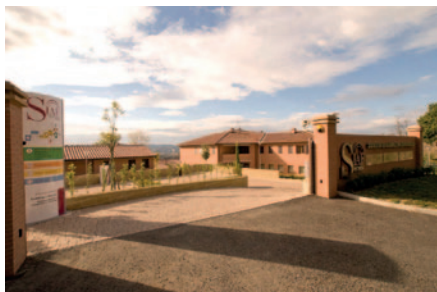
Venue for the 'Regional Development Agencies: The Next Generation Networking, Knowledge and Regional Change' workshop
