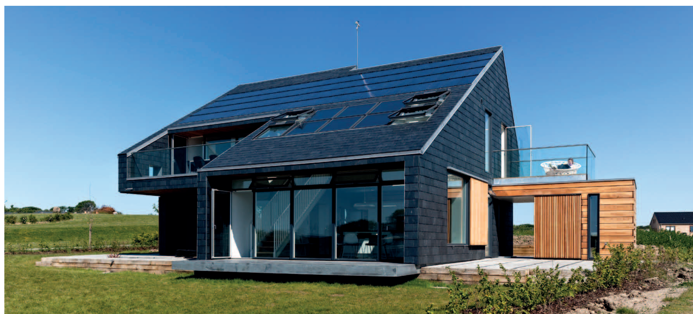
"Home for Life". South facade
