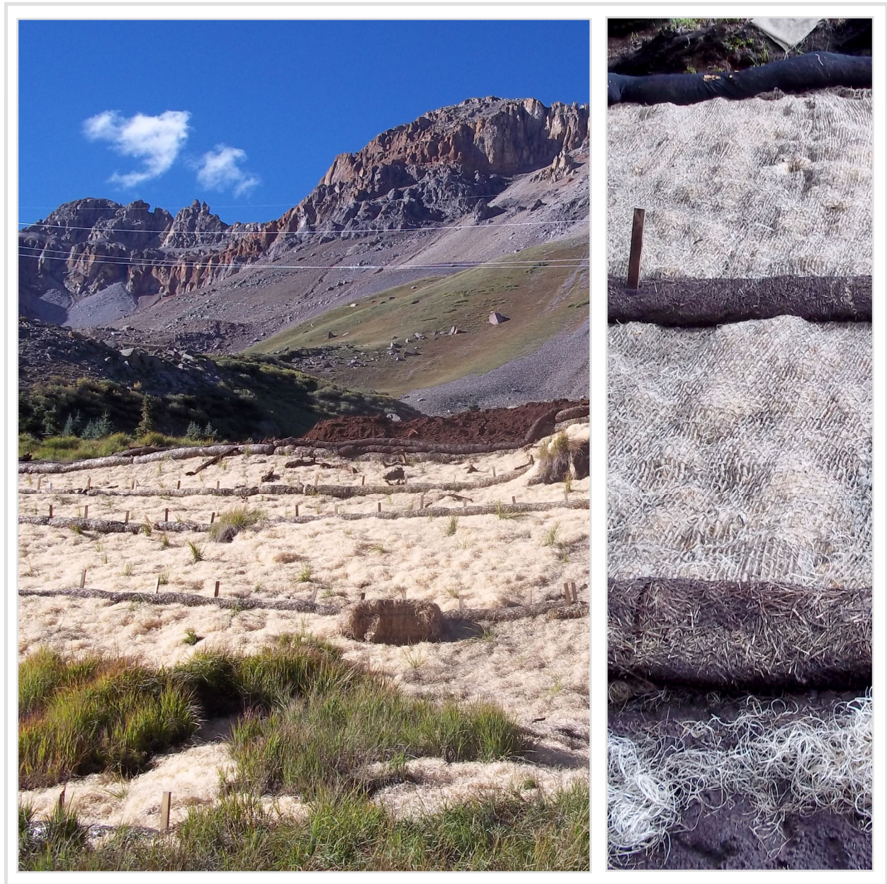
Figure 39. Example of erosion control on a steep mountain fen in Colorado. The slope is initially covered with mulch (left), followed by jute matting, and straw wattles are placed to reduce water flow (right).
