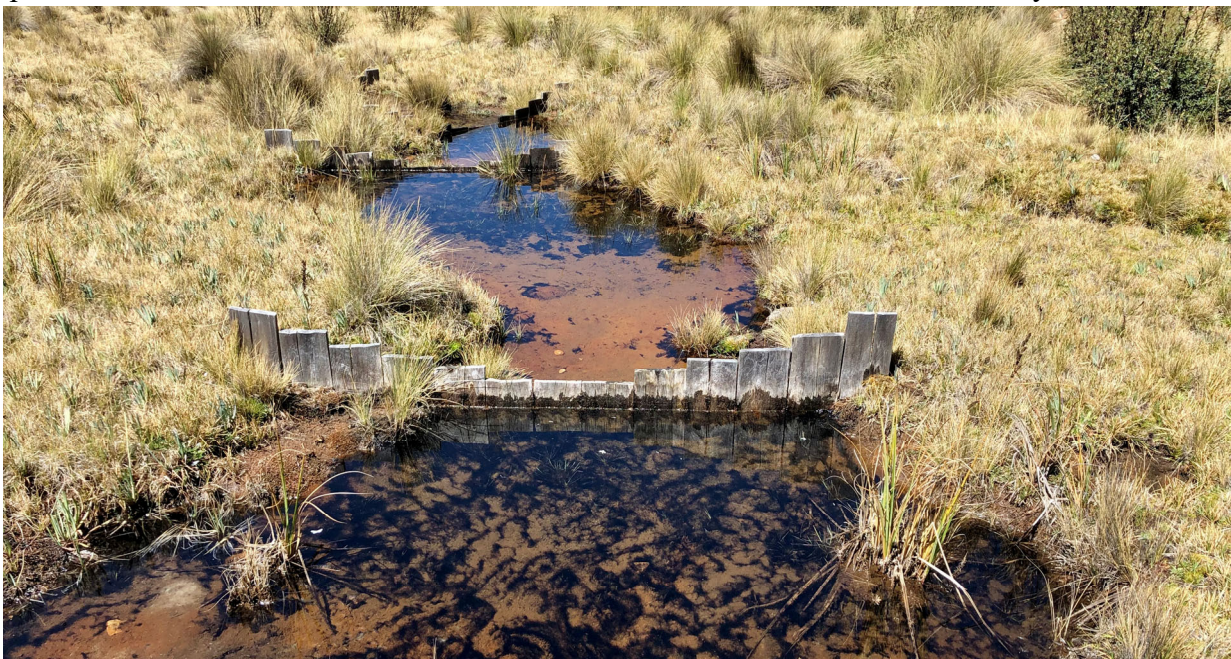
Figure 30. Example of ditch dam spacing by placing dams in a location that when the water backs up from the bottom dam the ditch is filled with water to a level above the base of the next dam up slope.
