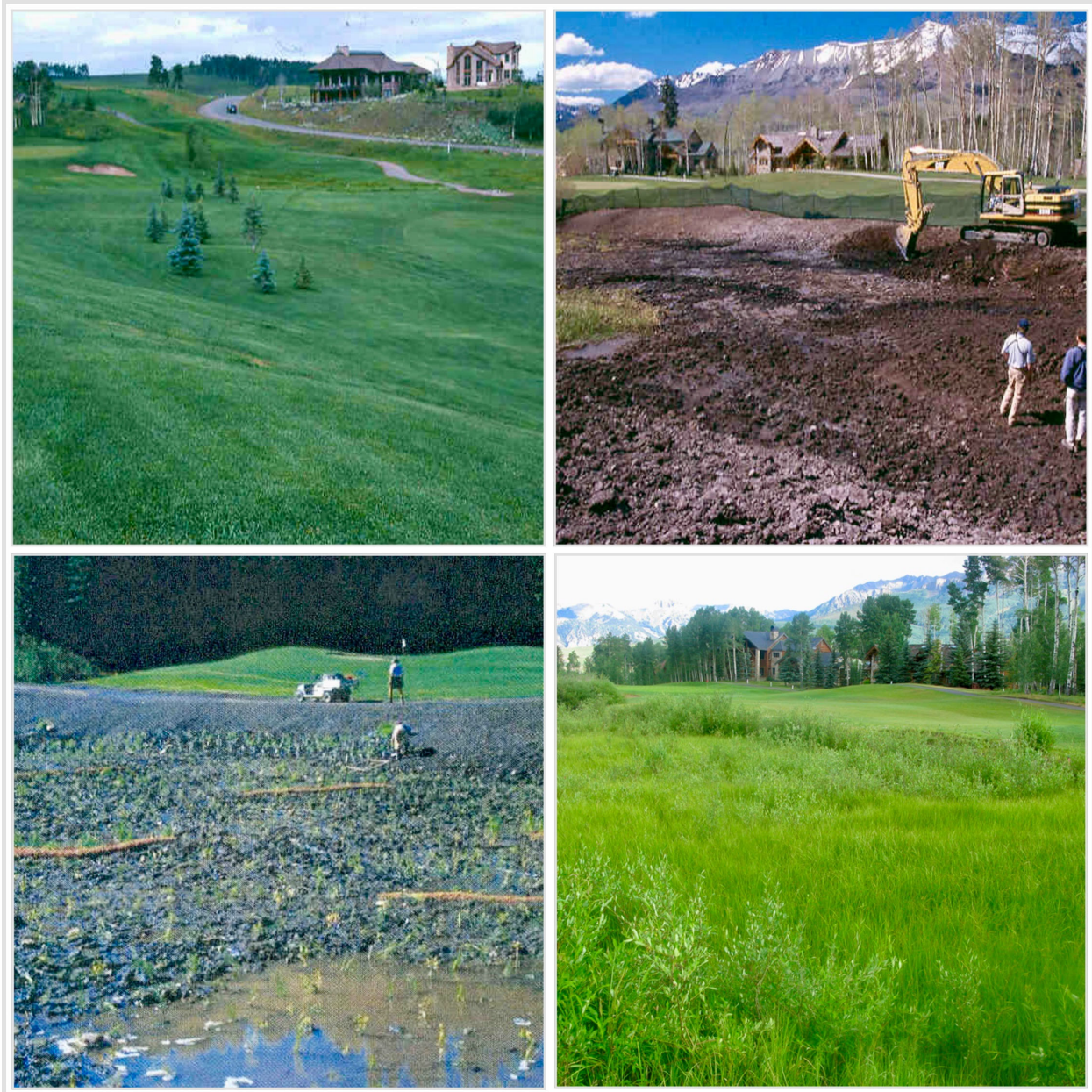
Figure 37. Sequence of photos showing a golf course that was built on top of a fen (top left), excavation of fill from golf course (top right), revegetation of excavated fen (bottom left), and restored fen (bottom right).
