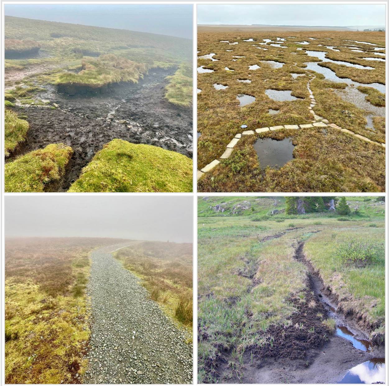
Figure 42. Peat erosion from hiking across a mountain peatland in Wales (top left), new gravel trail built across the peat in Wales (bottom left), flagstone walking path in Scotland (top right) and vehicle tracks in a Colorado fen that are at least 15 years old and initiated a small gully (bottom right).
