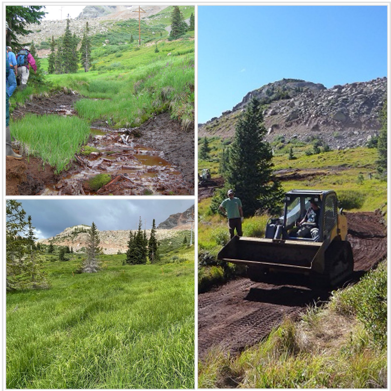
Figure 19. Example of filling in a ditch with native peat. Ditch before restoration in 2007 (top left), during restoration in 2012 (right), and after restoration 2023 (bottom left).
