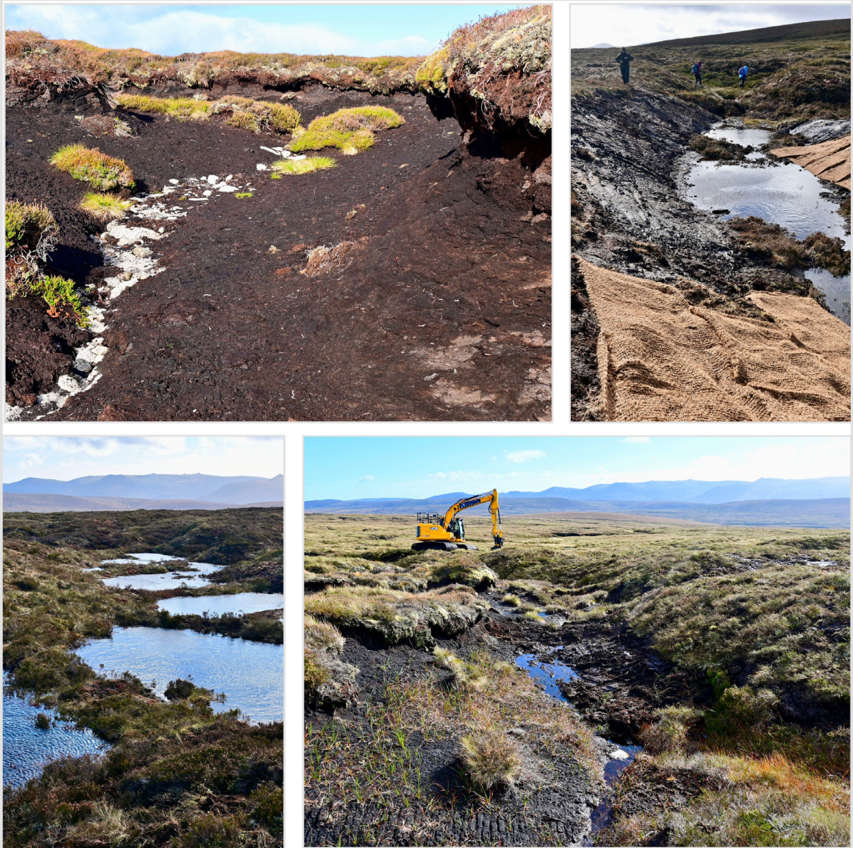
Figure 35. Gully reprofiling in Scotland. A gully causing peat erosion and drying (top left), gully reprofiling with an excavator (bottom right), steep side walls covered with coir matting and planted (top right), and restored gully (bottom left).
