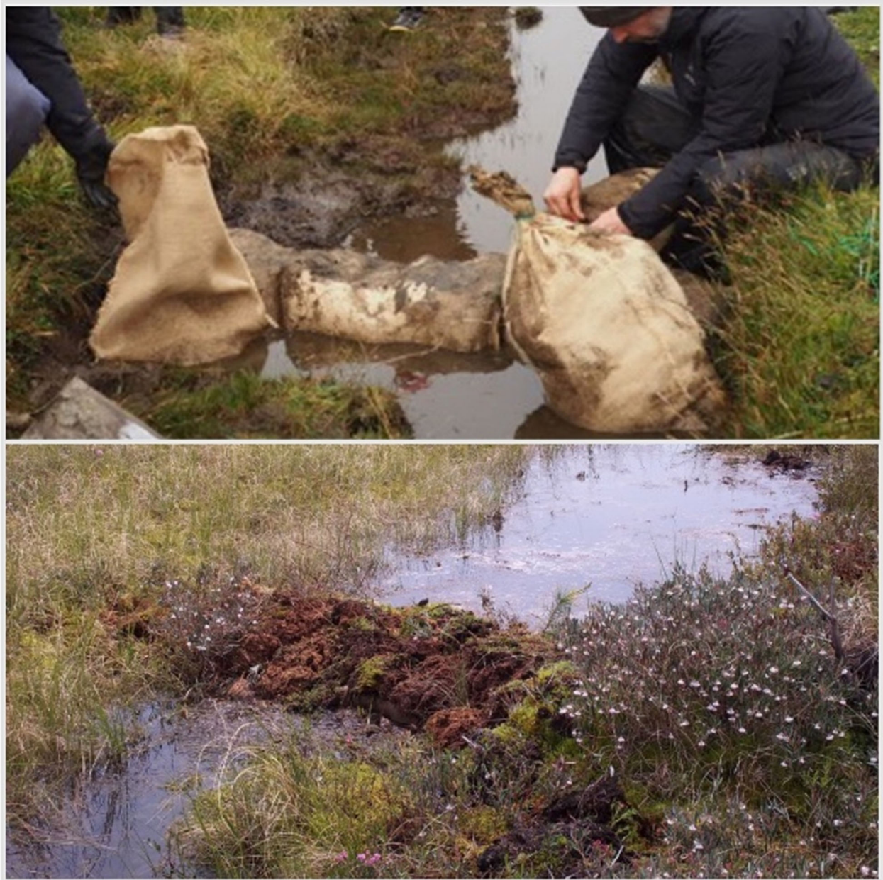
Figure 25. Example of using bags to create living impermeable ditch dams for low flow ditches. Filling and placing jute bags in bottom of ditch (top), then placing peat sod on top of bags (bottom).
