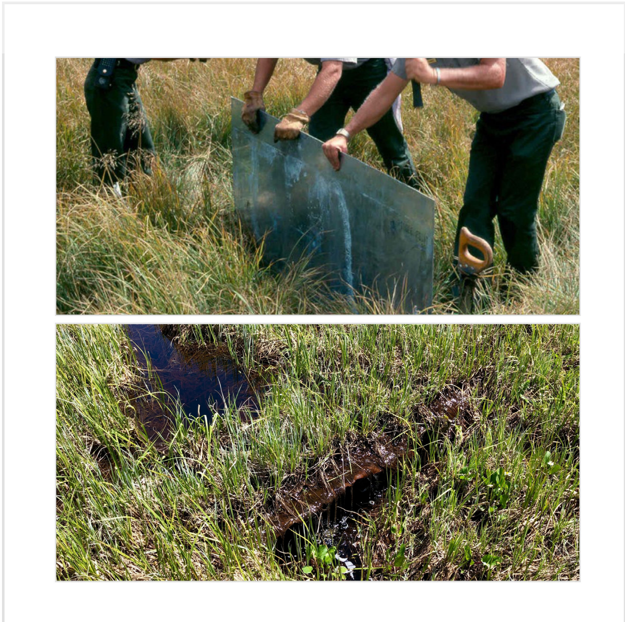
Figure 28. Steel dams installed (top) in 1988 and their condition 33 years later (bottom).
