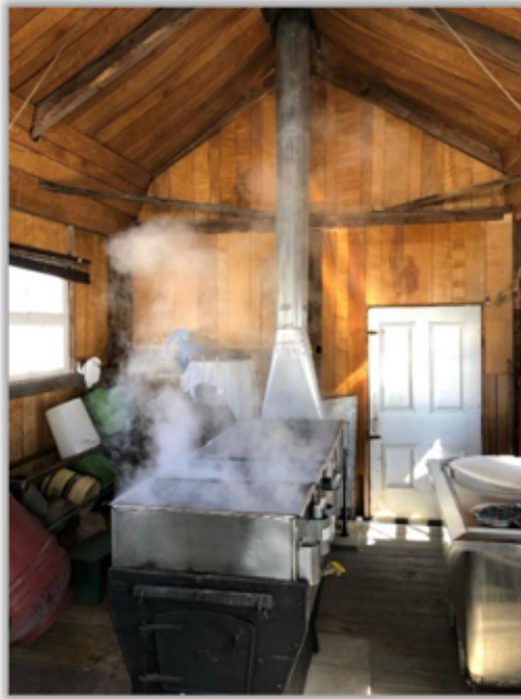
Wood-burning evaporator with three main compartments.
