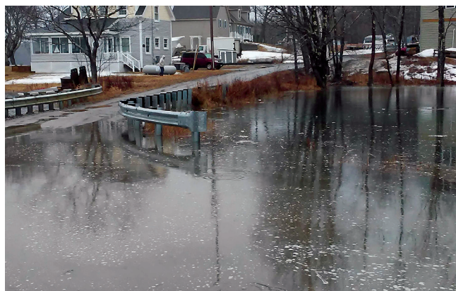
FIGURE 2: Flooding during a King Tide in Harpswell
