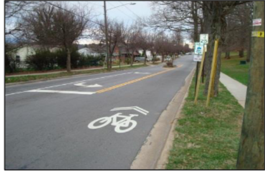
Figure 32: Shared Lane Marking
