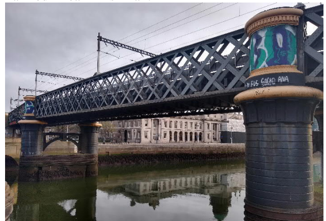
Figure 1. The Loopline Bridge span over the River Liffey.
