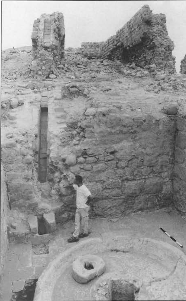
11. View of two parallel oblique penstocks from north-eastern edge-runner water mill chamber in Trench VI, Ṭawāḥin as-Sukkar (photo: K. D. Politis).
