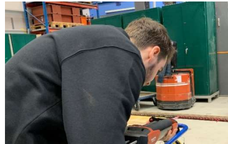
Figure 18: Installation process of the FOS on reinforcement steel bars
