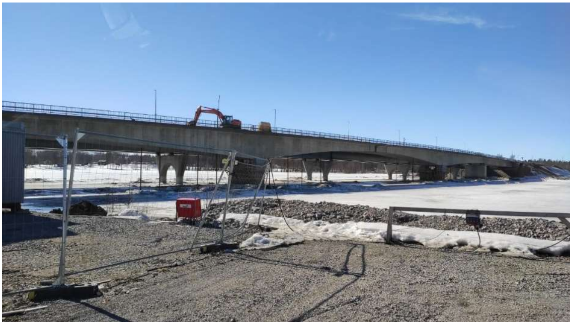
Figure 34: The 65 years old bridge situated in Kalix (Northern view)
