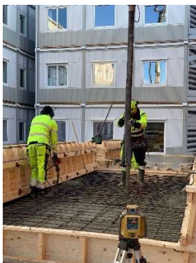
Figure 11: Casting Day; Trough bridge #1 being cast
