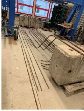
Figure 15: Reinforcement bars for cast trough bridges
