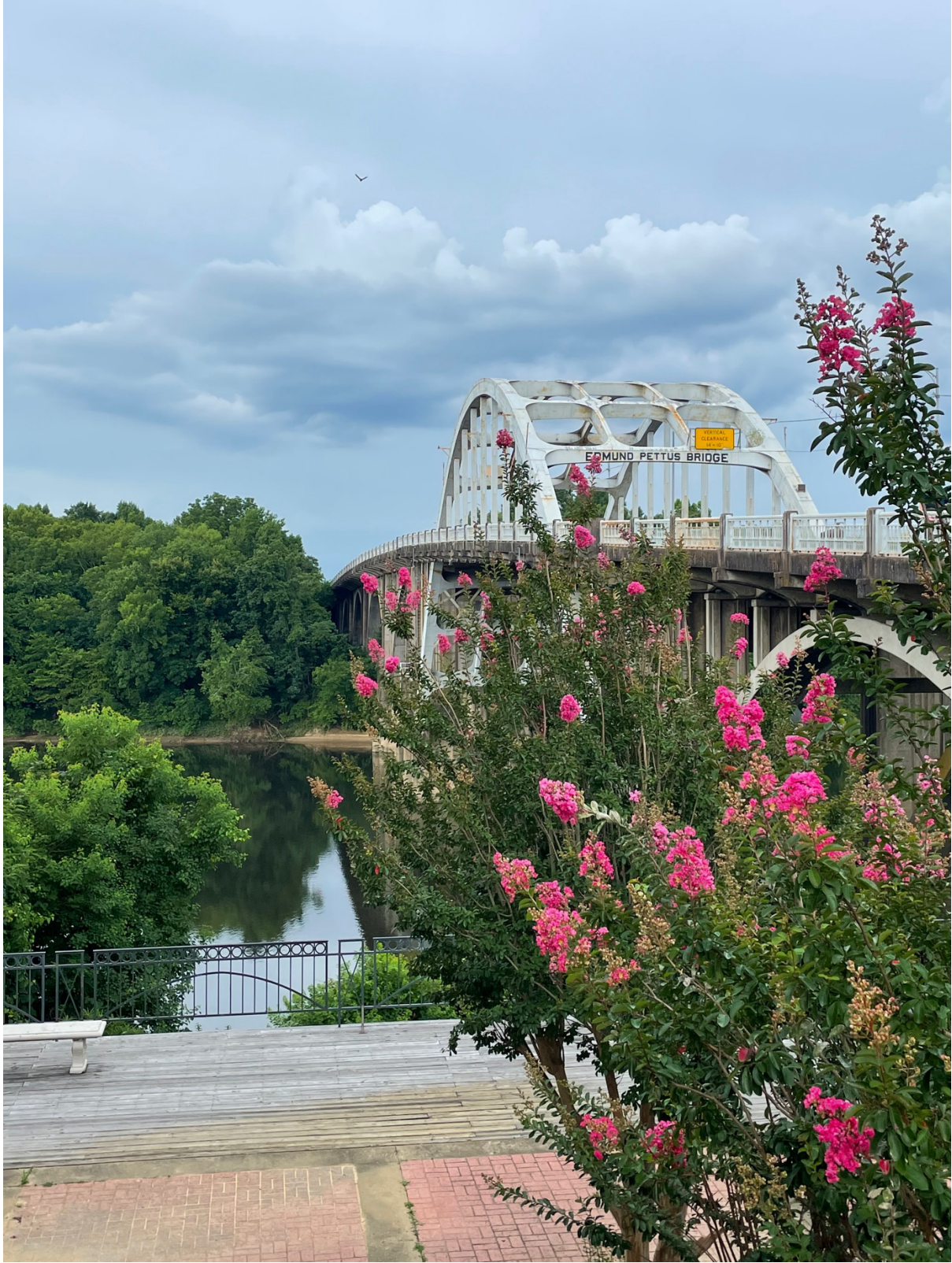
The Edmund Pettus Bridge – Selma, Alabama. Photo: Allyson K. Hayden, June 29, 2022.
