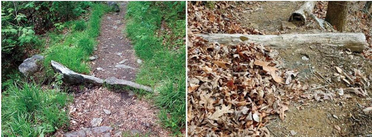
Figure 4. Examples of trail drainage features made of stone (left) and wood (right) (U.S. National Park Service).
