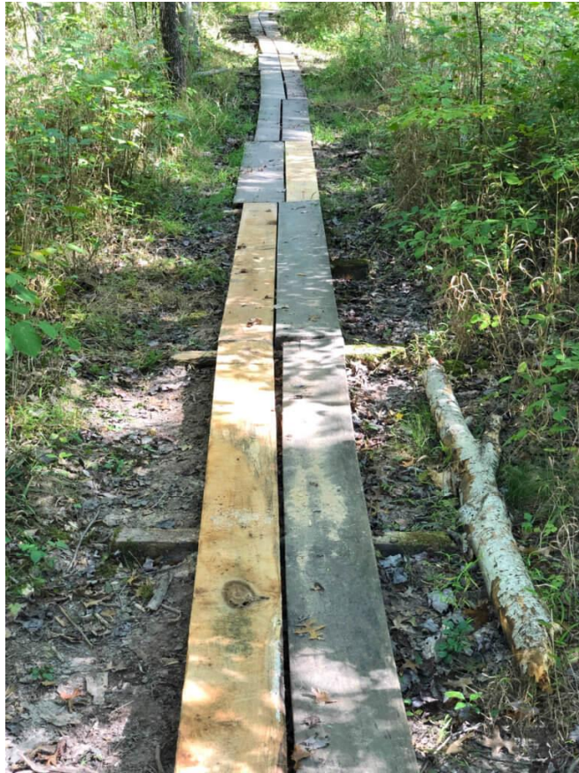
Figure 5. An example of a puncheon boardwalk mirroring the structure of the boardwalks planned for construction in Turtle Creek Park.
