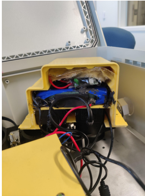
Figure B1. Picture of the right side of the electrical components: houses the batteries for the system.
