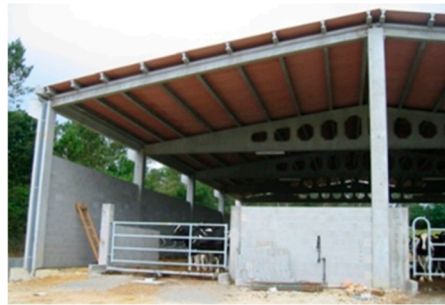
Figure 1. A typical concrete dairy farm showing pillars and beams.
