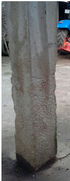
Figure 2. An image of a pillar showing typical deterioration by aggressive environment. Notice the loose of section in the lower part.
