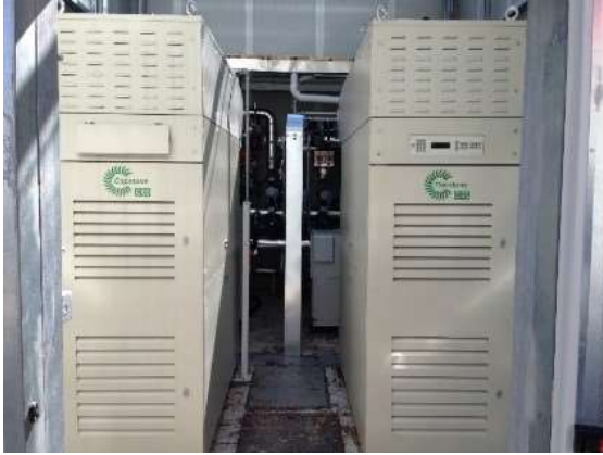
Figure 3.2. Microturbines (left) and one boiler (right) of the SPM [32].
