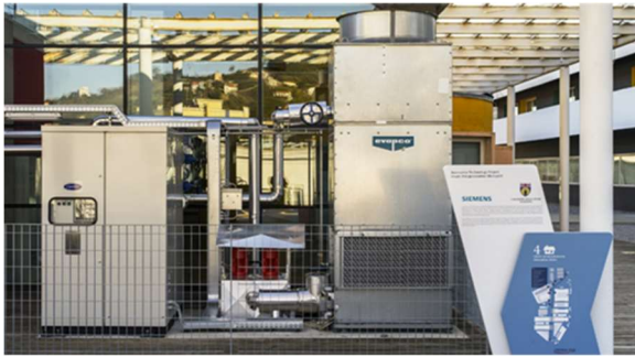
Figure 3.3. Absorption chillers of the SPM [32].
