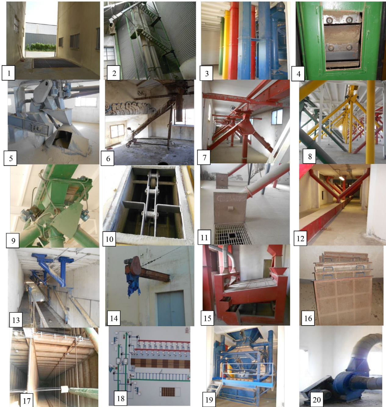
Figure 3. 1) Reception hopper in type J silo at Corrales del Vino, Zamora; 2) grain elevator in type MC silo at El Pedroso de la Armuña, Salamanca; 3) grain elevators in type TV silo at Zuera, Zaragoza; 4) detail of elevator scoop in type TH silo at Medina del Campo, Valladolid; 5) circular distributor in type B silo at Villafranca de los Barros, Badajoz; 6) portable loading tube in subtype D 1 silo at Piedrahita de Castro, Zamora; 7) upper horizontal belt conveyor and loading tubes in subtype D 5 silo at Manganeses de la Lampreana, Zamora; 8) load tubes in type TV silo at Coscurita, Soria; 9) detail of damper and bypass valves in type TV silo at Coscurita, Soria; 10) detail of drive chain and crossbars inside upper horizontal belt conveyor in type TV silo at Coscurita, Soria; 11) loading tube and cell in type J silo at Cella, Teruel; 12) offloading tubes and lower horizontal belt conveyor in type J silo at Santa Eulalia del Campo, Teruel; 13) telescopic offloading tubes in type TV silo at Barcial del Barco, Zamora; 14) external bulk offloading tube in subtype D 4 silo at Herrera de Pisuerga, Palencia; 15) cleaning machinery in Type E silo at Lora del Río, Seville; 16) detail of cleaning screens in type TV silo at Coscurita, Soria; 17) interior of steel cells in type MR silo at Palanquinos, León; 18) control panel in subtype TR 5 silo at Medina de Rioseco, Valladolid; 19) automatic scales in type TH silo at Medina del Campo, Valladolid; 20) dust collector in type TE silo at Cariñena, Zaragoza; 21) dust filter in type TE silo at Cariñena, Zaragoza; 22) dust extraction chimneys in type SV silo at Badajoz; 23) thermometric sensors in type TH silo at Medina del Campo, Valladolid; 24) refrigeration facility in type TH silo at Medina del Campo, Valladolid; 25) lift in type TE silo at Pancorbo, Burgos; 26) intercom in type TV silo at Osma La Rasa, Soria; 27) lift to access cells for cleaning in type TE silo at El Carpio (Córdoba).
