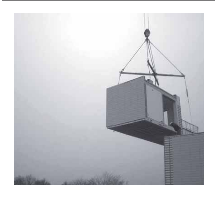
Complete volume-element being craned in place on site, Boel Living, fall 2007 .
