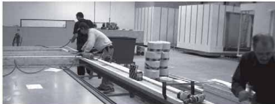
Figure 3: Traditional Wood-frame Construction in Production at Boel Living
