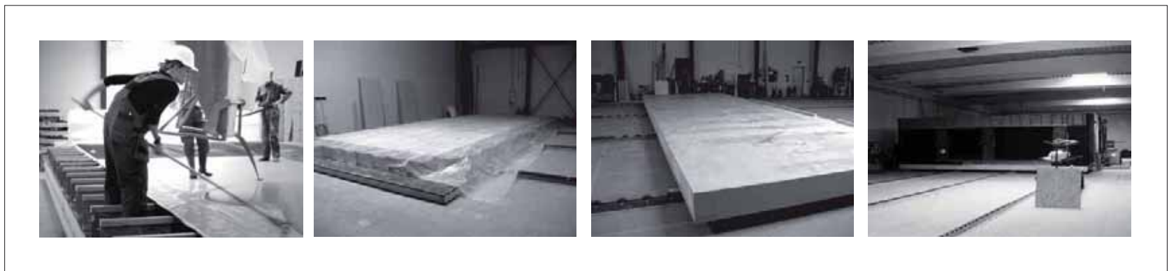
Casting of comple 4500 x 12500 mm deck-element summer 2009
