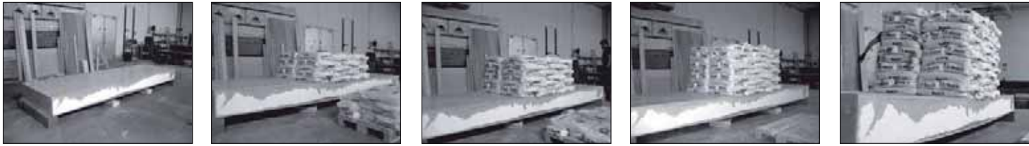
Test of bending strength of the high-strength concrete and EPS sandwich, spring 2009
