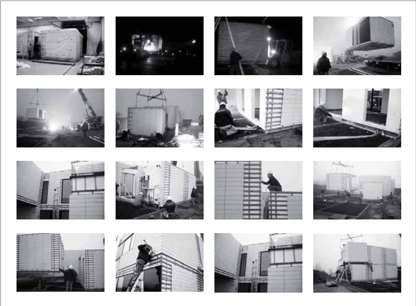
Production research at Boel Living, transportation and on-site assembly of complete volume-elements, fall 2007.
