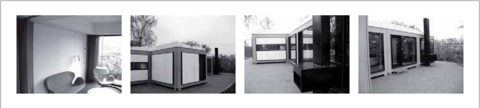
Prototype of Arne Jacobsen's 'Kubeflex' prefab house consisting of cubic volume-elements designed in 1971.
