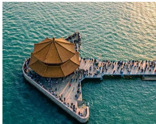
Fig. 4. Qingdao Trestle Bridge
