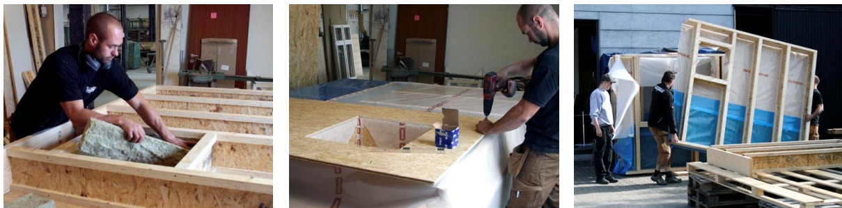
FIG 1. Construction of the new building façade in a controlled environment.
