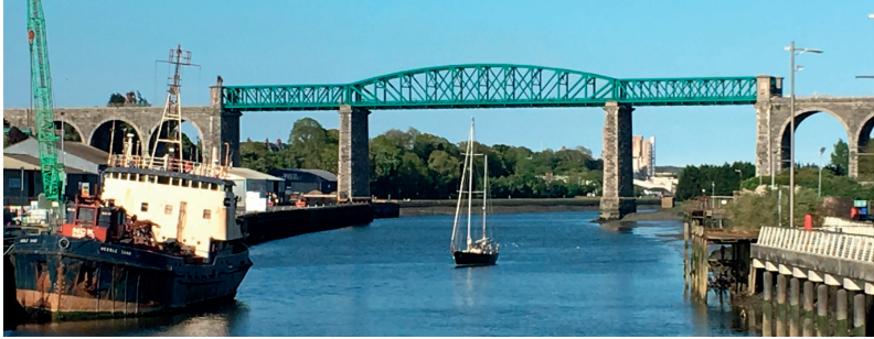
Figure 3.20: The Boyne Viaduct railway bridge in Drogheda, Ireland
