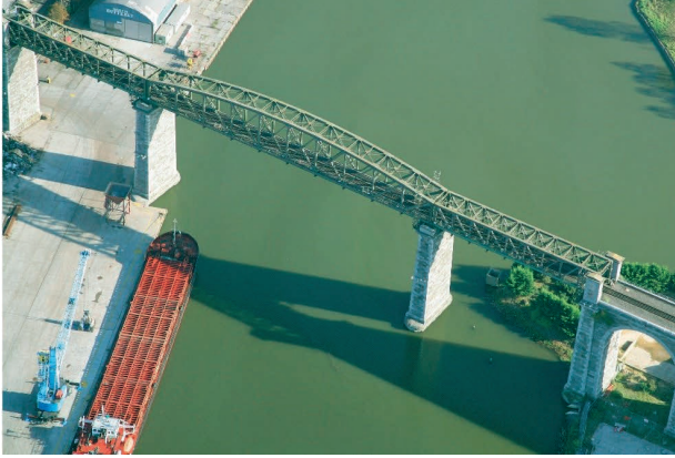
Figure 2.6: Aerial view of the Boyne Viaduct superstructure
