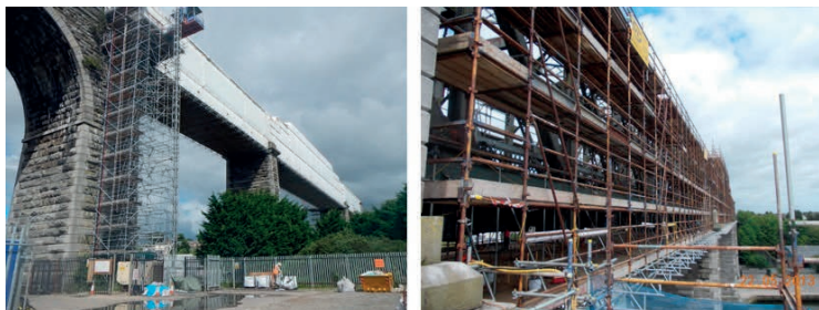
Figure 2.7: Scaffolding on the Boyne Viaduct
