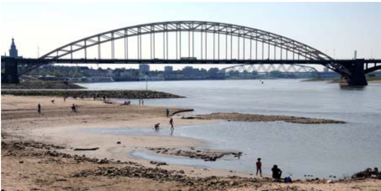
Figure 1: Low water levels at the Waal near Nijmegen. Photo © Ronald Puma.
