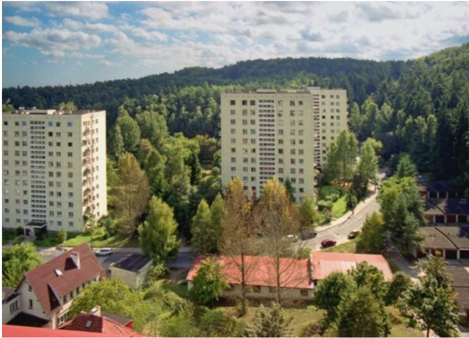
Figure 5.16. View of the WSM site, including buildings 57, 59 and 61 (from left to right). Photo by Czesław Piechnik, via WSM website ( www.wsmsopot.jimdofree.com ).
