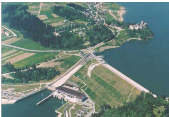
Fig. 1. The View of Czorsztyn-Niedzica dam.
