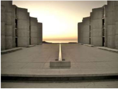
Figure 8 - Transforming a space through lighting, Salk Institute.
