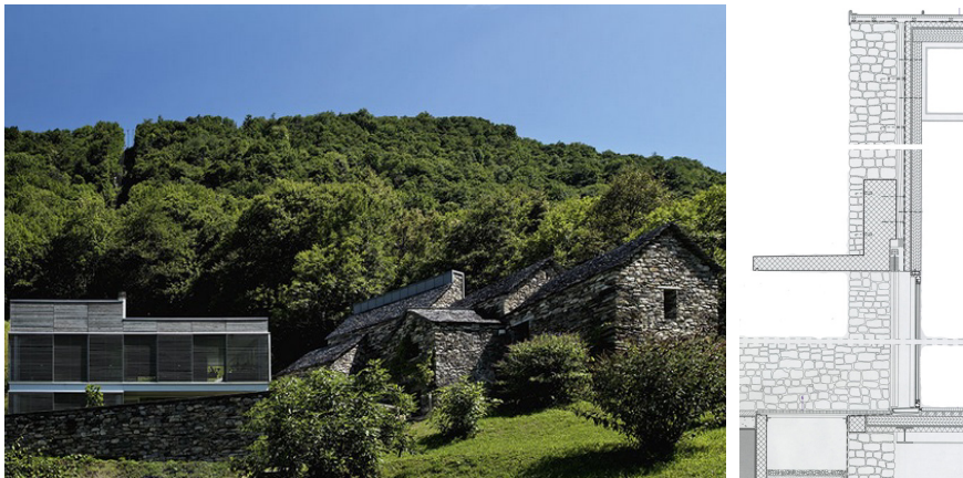
Figure 2: Pianezzo: village and construction detail of gneiss stone dwelling.
