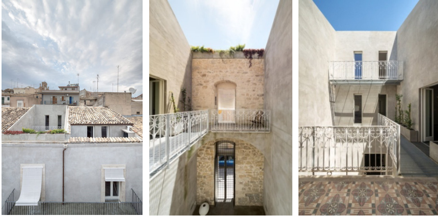
Figure 4: Ragusa: images of the recovered building.
