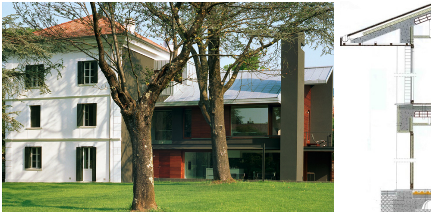
Figure 1: Tarcento: south façade and construction detail.
