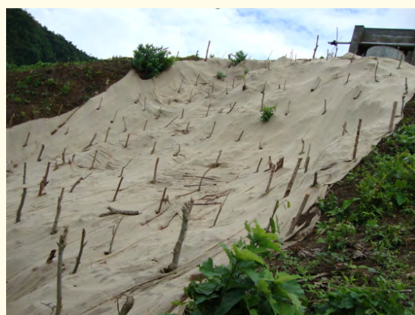
Figure 4: Reclamation of degraded sloping land by Geojute, Photo Credit: A. M. Zahid, SRDI.
